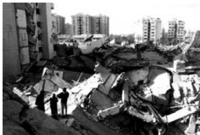
Residents of Ahmedabad, India, survey earthquake damage. (AP Photo/Saurabh Das)
